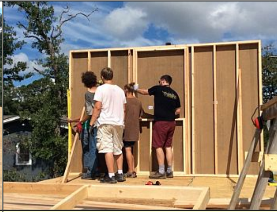
The walls on the 2nd floor are going up!
