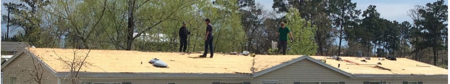
**Once all the repairs are made the roof is ready to be cleared for a new covering.**
